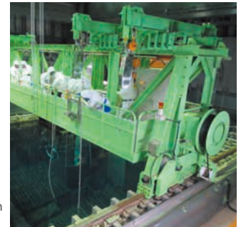
Removing fuel from the SFP
