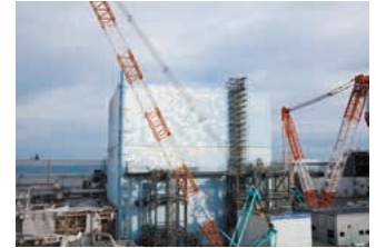
Installation of a working platform
